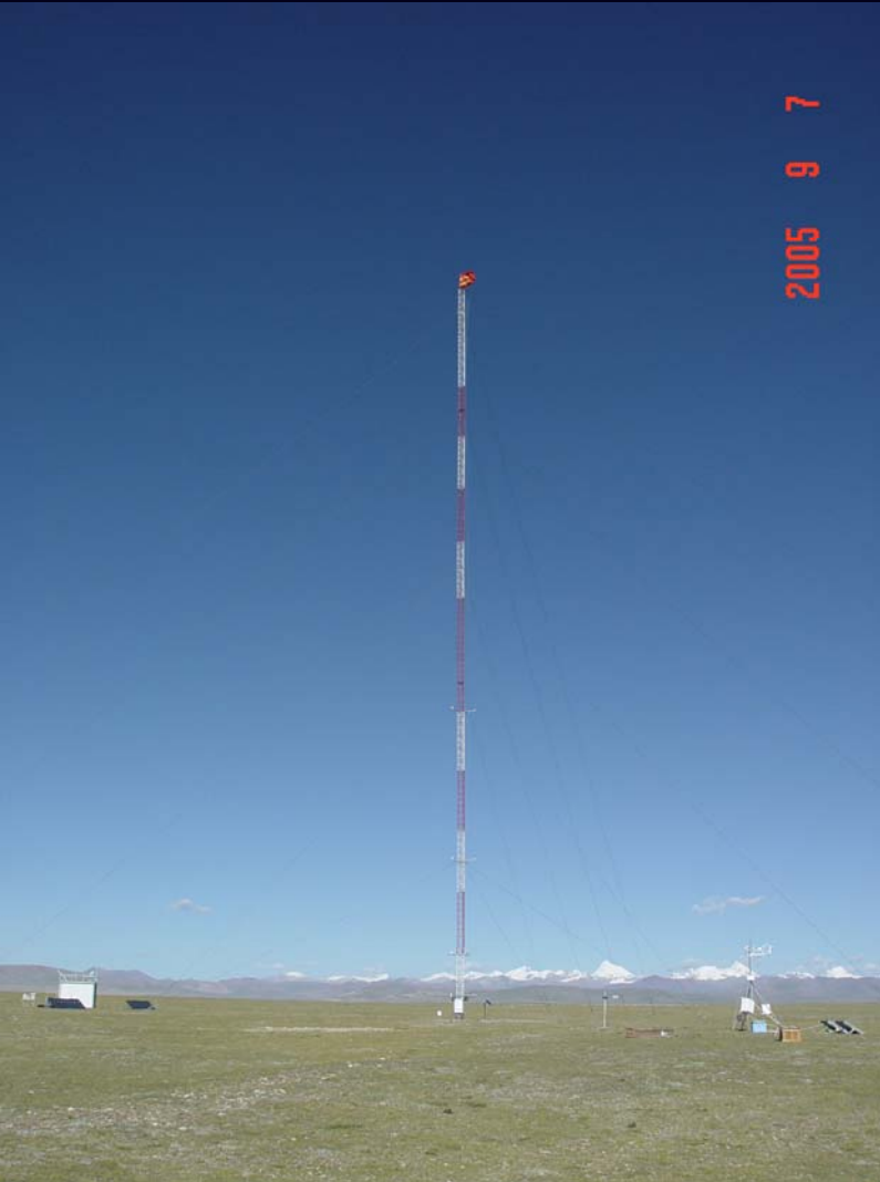
52m PBL tower ( Radiation system and SMTMS)
